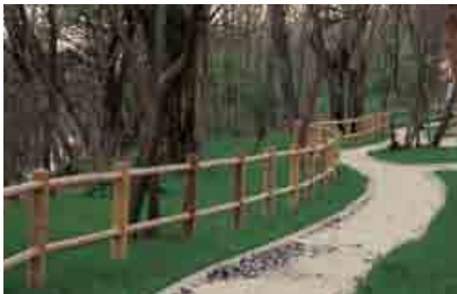
Interasse 2000/2500 mm Montanti Ø 120 mm o Ø 140 mm Traversi Ø 80
